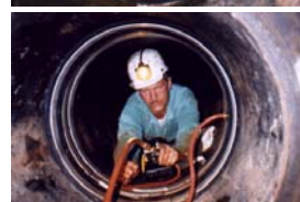
Pressure Test Seal
