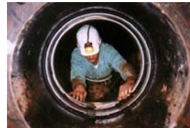
Install Retaining Bands
