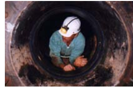
Install Rubber Seal
