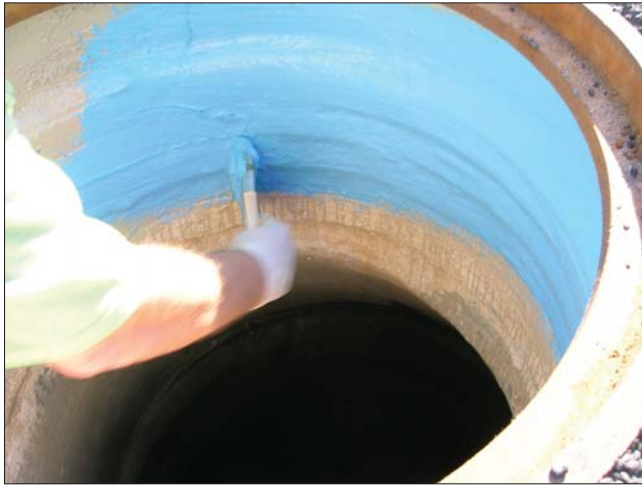
A urethane internal seal is applied to a manhole chimney. The finished project is at the right.
