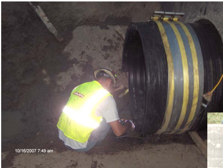
PREPARING 42 inch HDPE PIPE WITH CENTERING BAND
