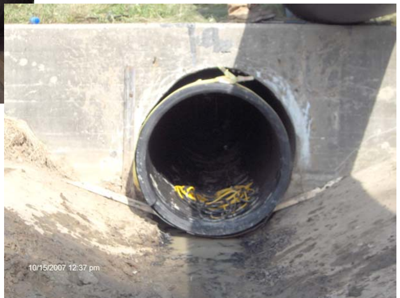
42 inch HDPE INSERTED INTO 54 inch CMP
