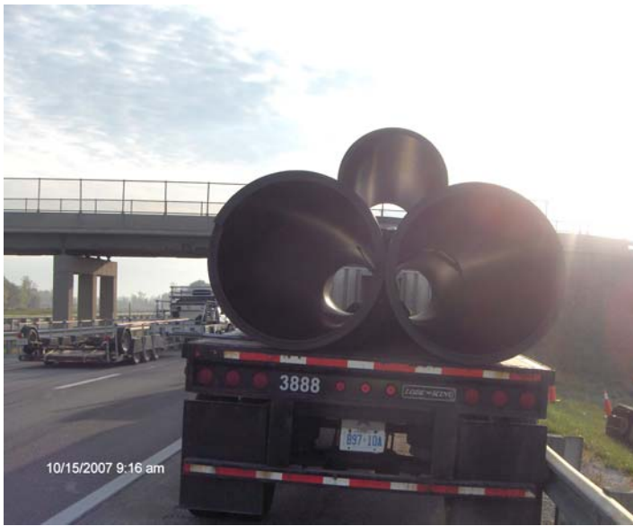
20 foot LENGTHS OF 42 inch HDPE PIPE ARRIVING AT JOB SITE
