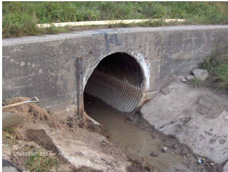
EXISTING 54 inch CMP PIPE
